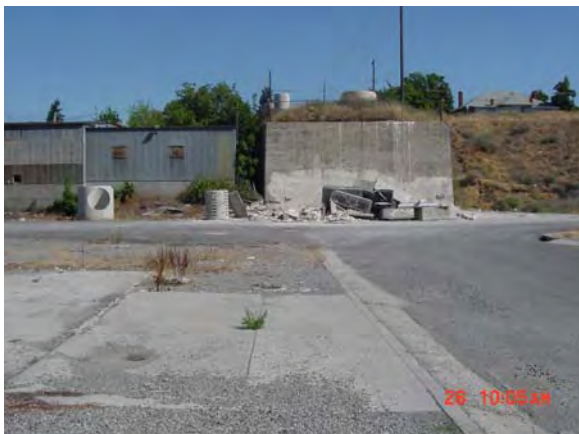
View of bluff and cement bridge abutment. Roof of residential home can be seen in top right. July 2001
