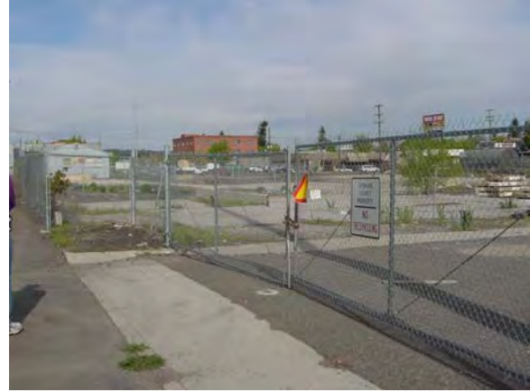
View of site after buildings were demolished. The only structure remaining is the gray structure on the center left. May 2003.
