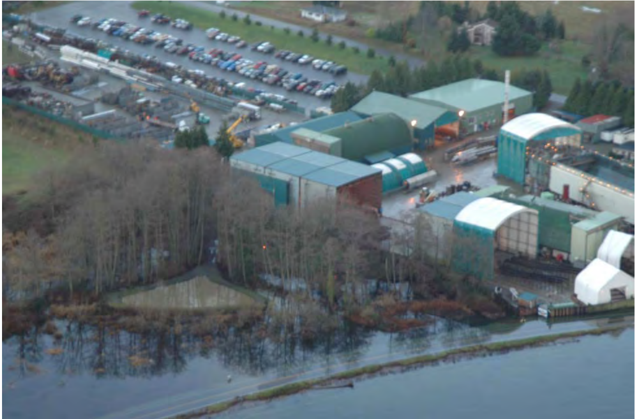
Photo 2. Southwestern Shore of Holmes Harbor during high tide, showing the infiltration basin for NBBBI wastewater and storm water
