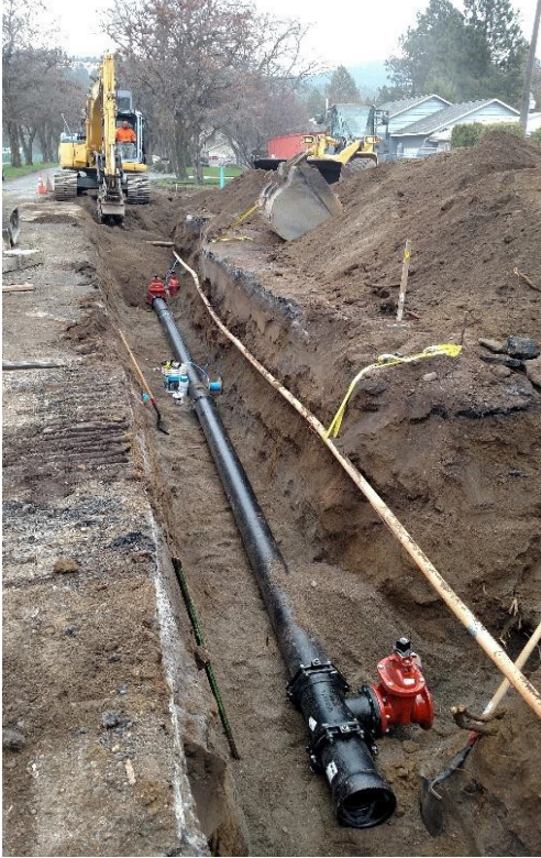
Installation of new water main.
