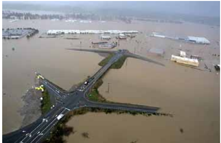
The December 2007 floods completely submerged Interstate 5 in Lewis County. Flooding damaged several area water systems. (Photo courtesy of Washington Department of Transportation.)
