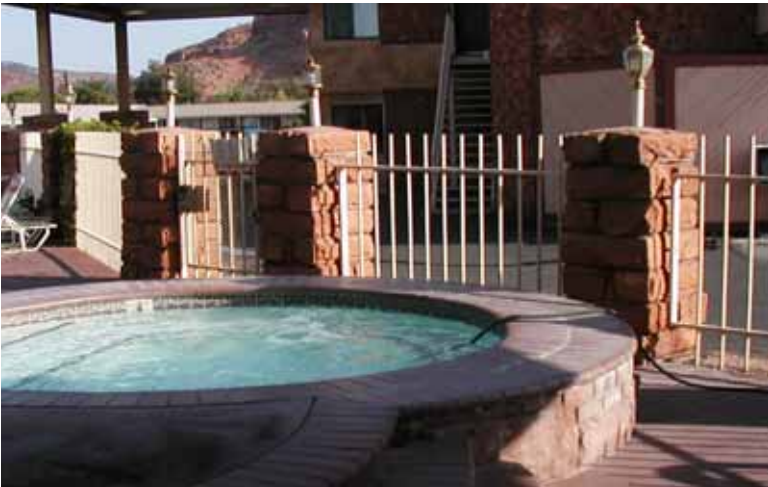
Hose-end immersed in water with no air gap creating a cross-connection hazard
