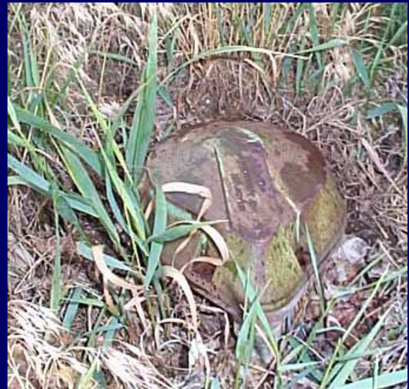
Well Casing terminating close to ground surface.
