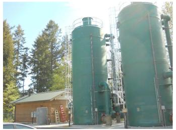
Packed tower aeration facility for corrosion control.
