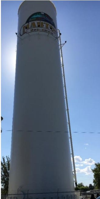
New 1-million-gallon reservoir
