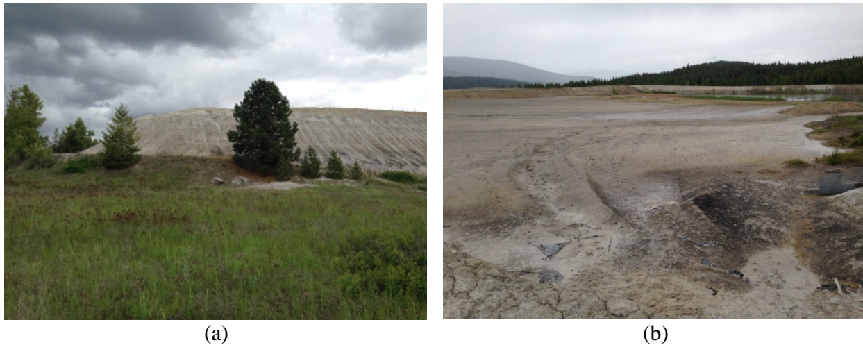
Figure 4: Lower Tailings Pile (a) view from Van Stone Mine Road and (b) view from top of pile, Van Stone Mine, Stevens County, WA (May 29, 2014)
