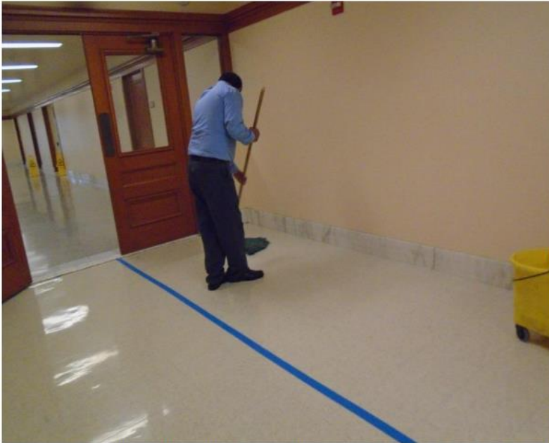
Figure 2-11. Applying Alternative Stripper during Testing at San Francisco City Hall
