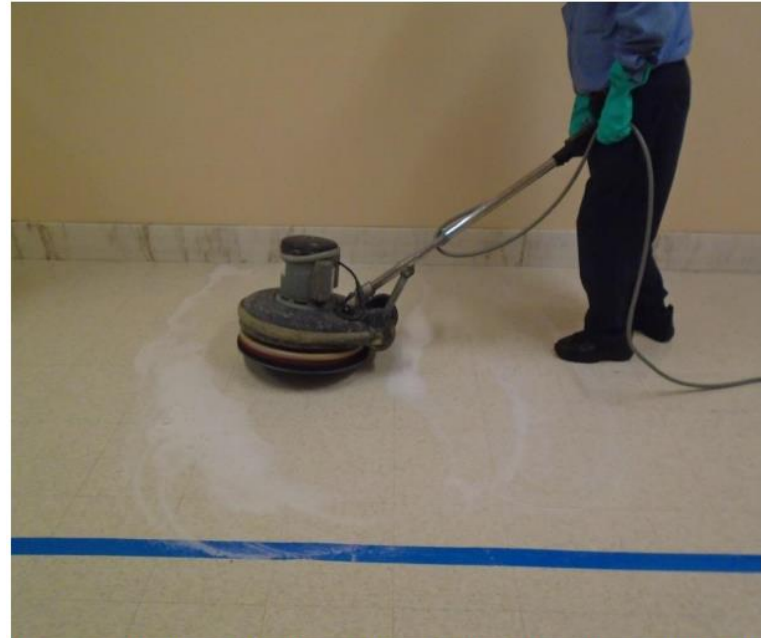
Figure 2-12. Using Floor Machine on Stripper during Testing at San Francisco City Hall
